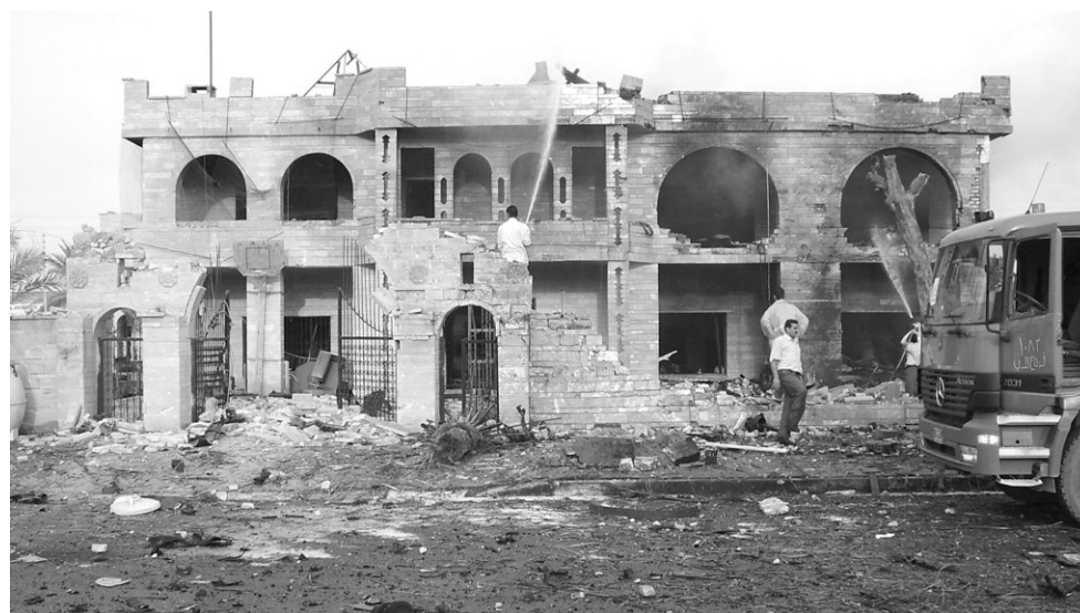
Photo taken less than 30 minutes after the explosion, in which the house was destroyed. The 3rd floor was completely gone, as there was a fighting position there with rockets and ammo that cooked off and blew up when the fire started.
